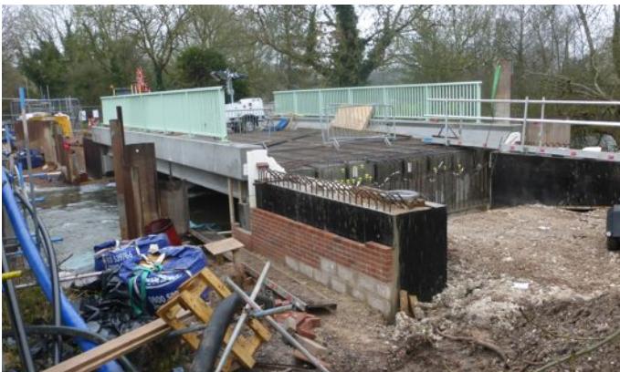
New Bridge Construction 2016
